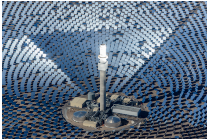
Figure 2 Crescent Dunes Power Tower. Note cylindrical molten salt thermal storage tanks at bottom center. Source: SolarReserve.
