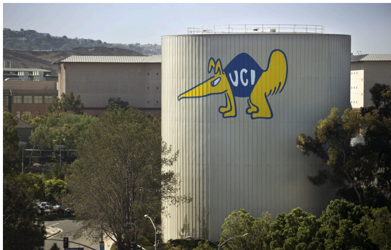
Figure 5 University of California Irvine chilled water storage, provides 65% of air conditioning (~74 MWh) load from power consumed at night. Source: Steve Zylius, UCI.
